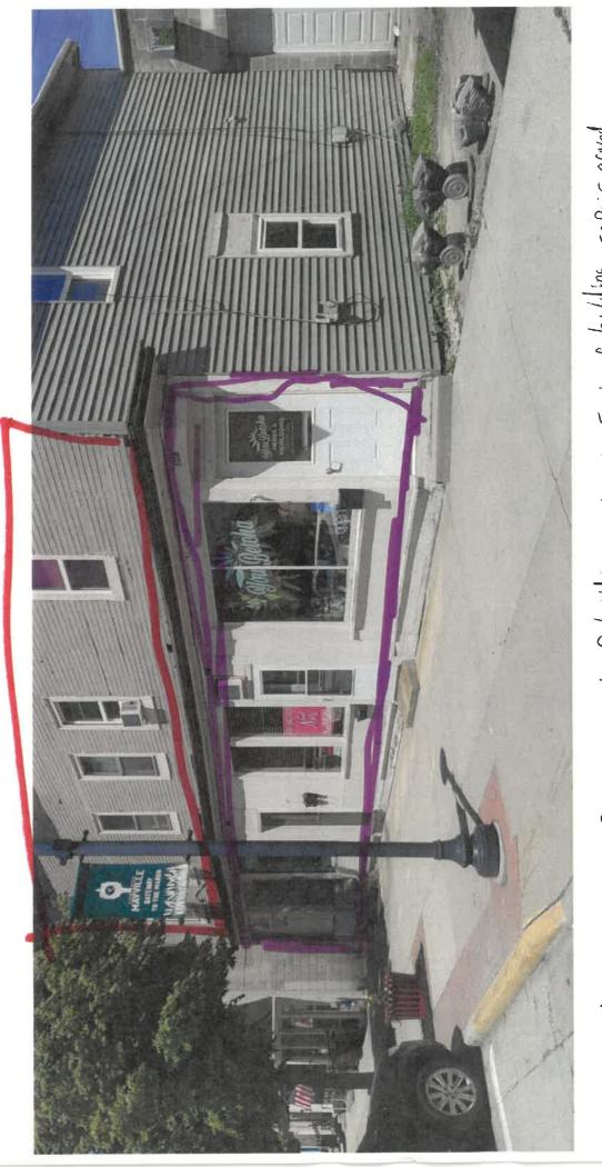
= Continue Vinyl Siding From South Side of building on the upper Front of building, repair around uns, and trim out alough.
