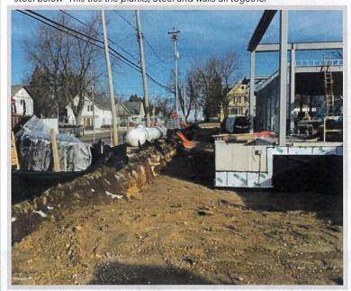
Above: Excavator is backfilling along the west foundation walls. Grade is close to the top of the concrete walls and once completely backfilled there will be easy access to complete the exterior skin of the building
