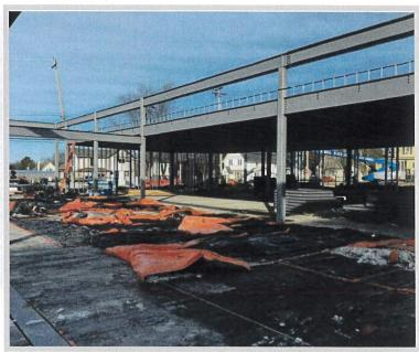
Above: Standing on precast deck, Steel has been set on the north half of the building and metal deck installed. Trusses will be set above this area and by this time next month the entire roof deck will be installed
