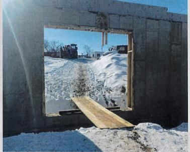
Above: This opening is the last portion of concrete walls to get poured. This was left open so equipment and material can be brought into the basement. Once the basement slab is poured, this wall will be filled in
